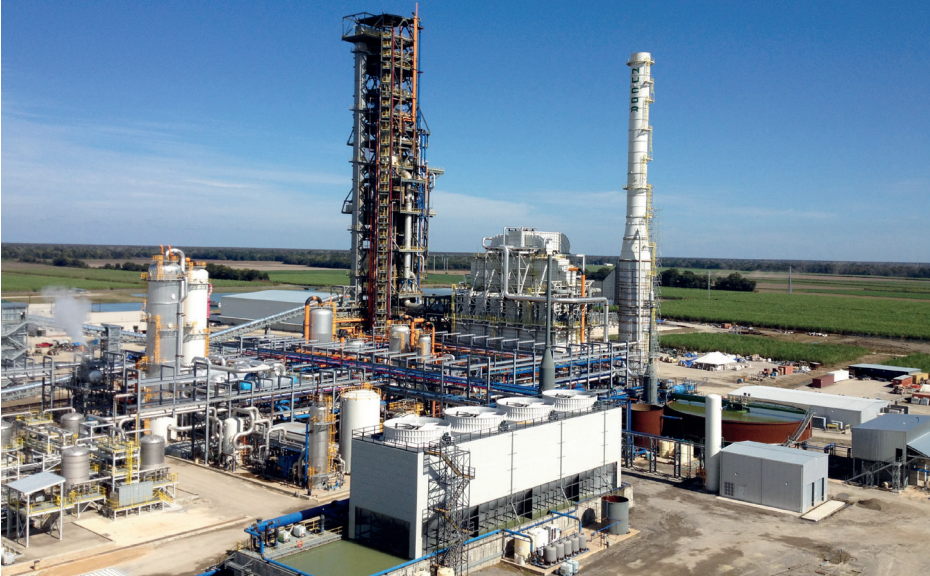
Picture 2. Nucor ENERGIRON DR Plant at Nucor Steel, Louisiana, USA, which has achieved a worldwide record of combined 330 t/h productivity with DRI @96%Mtz & 3,3%C
