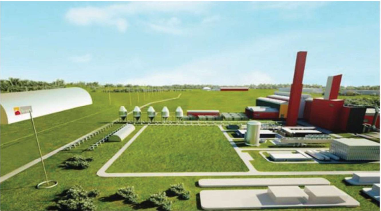
Fig. 6: Ternium Pesqueria Project including a 2.1Mtpy ENERGIRON DRI Plant
